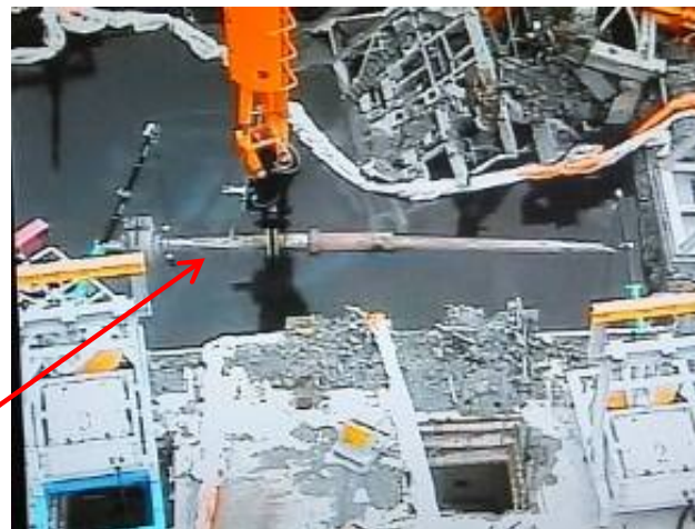
Removed fuel exchangers mast (3.27.2014)
