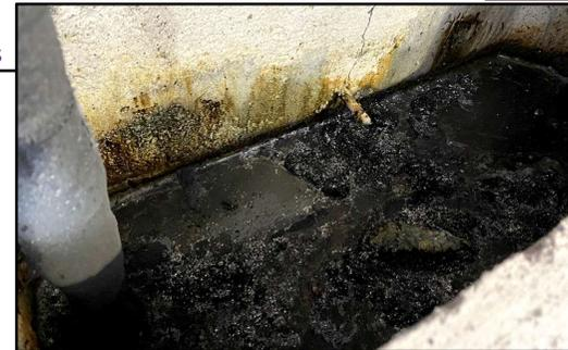
View into the melter showing the surface of the glass monolith.
